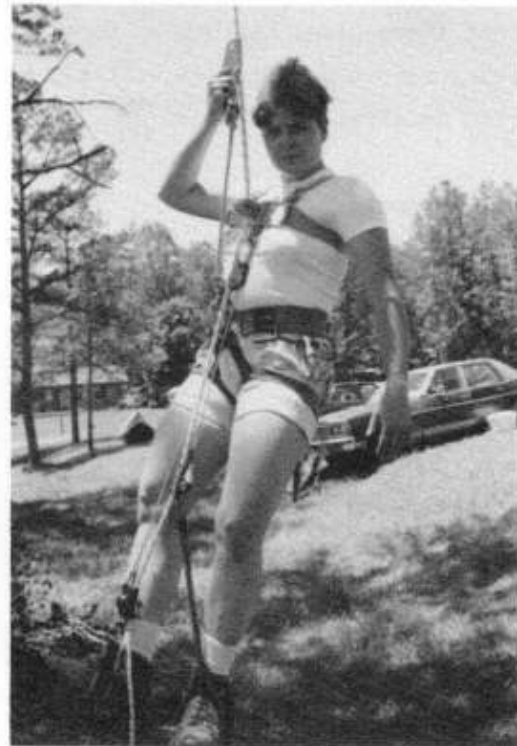
Full rig with safety running from the seat harness to the climber's right hand.
